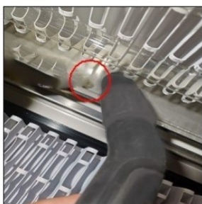
4. The dust inside the unit can be removed by a vacuum cleaner.
