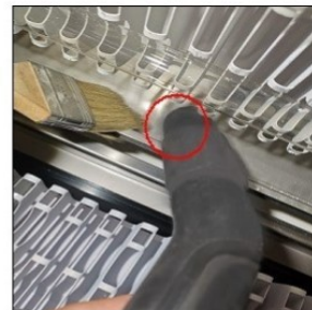
3. Hold the door and clean the UV lamps one by one and catalyst plates with a soft brush.
